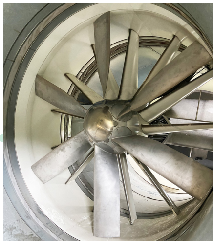
ZerAx® fan being installed
