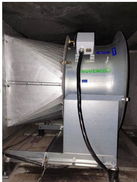
Horizontal or vertical installed in AHU, as for this large retrofit project, NOVENCO ZerAx EC+ fans efficiencies are consistently the highest available on the market
