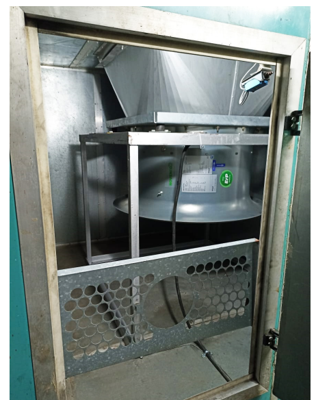
Horizontal or vertical installed in AHU, as for this large retrofit project, NOVENCO ZerAx EC+ fans efficiencies are consistently the highest available on the market
