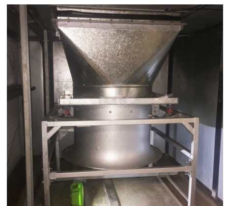
After retrofit - NOVENCO ZerAx EC+
